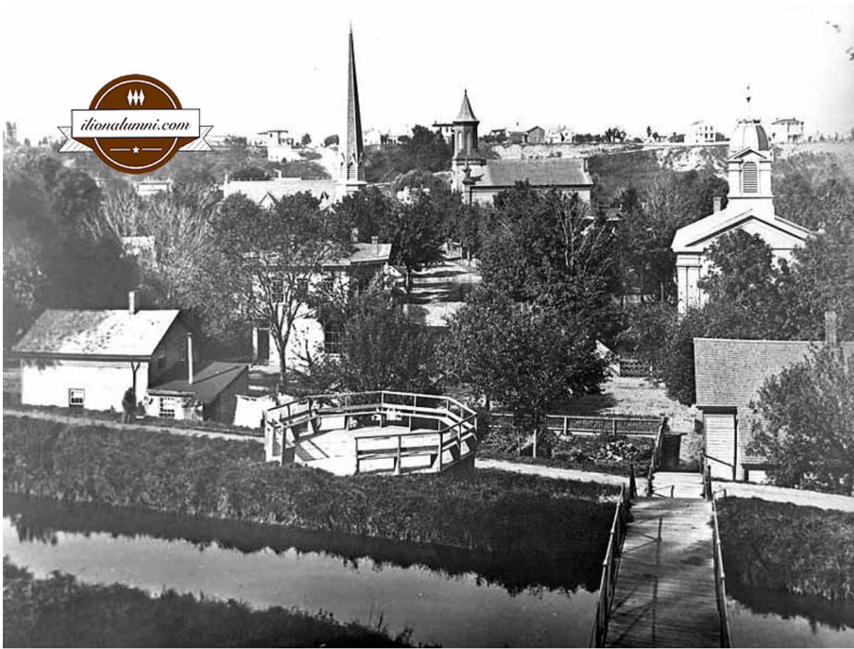
Armory Hill Steps pre-1896 - A footbridge covers the waterway to the Remington Arms
